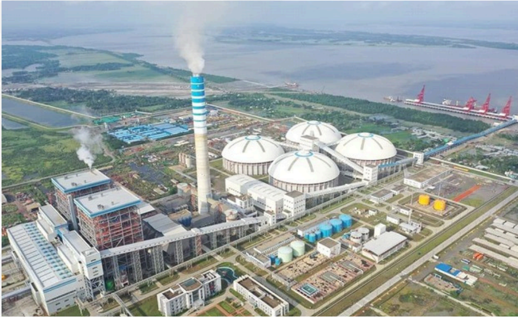
Payra Thermal Power plant
