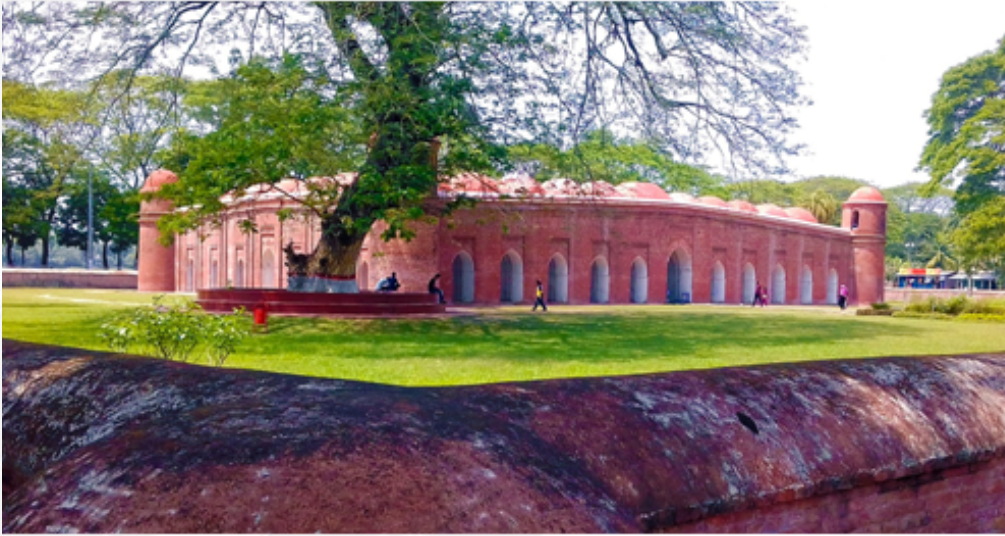
Sixty Dome Mosque, Bagerhat
